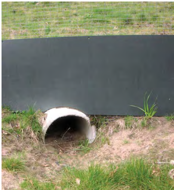
Figure C-8—Examples of small animal exclusion fencing (frogs, lizards, salamanders, toads, snakes, small mammals). Source: http://animexfencing.com/ ; Clevenger and Huijser 2011.
