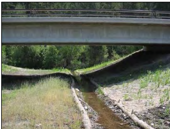
Figure C-3a—Bridge with channel that allows water to flow seasonally.
