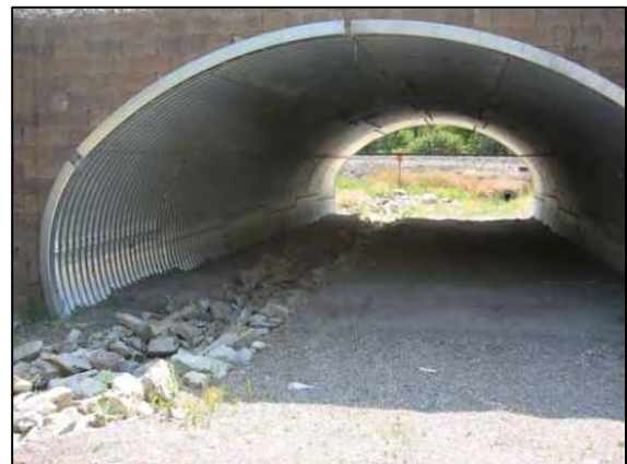
Figure C-3b—Arched culvert with a ditch on left that allows water to flow seasonally.
