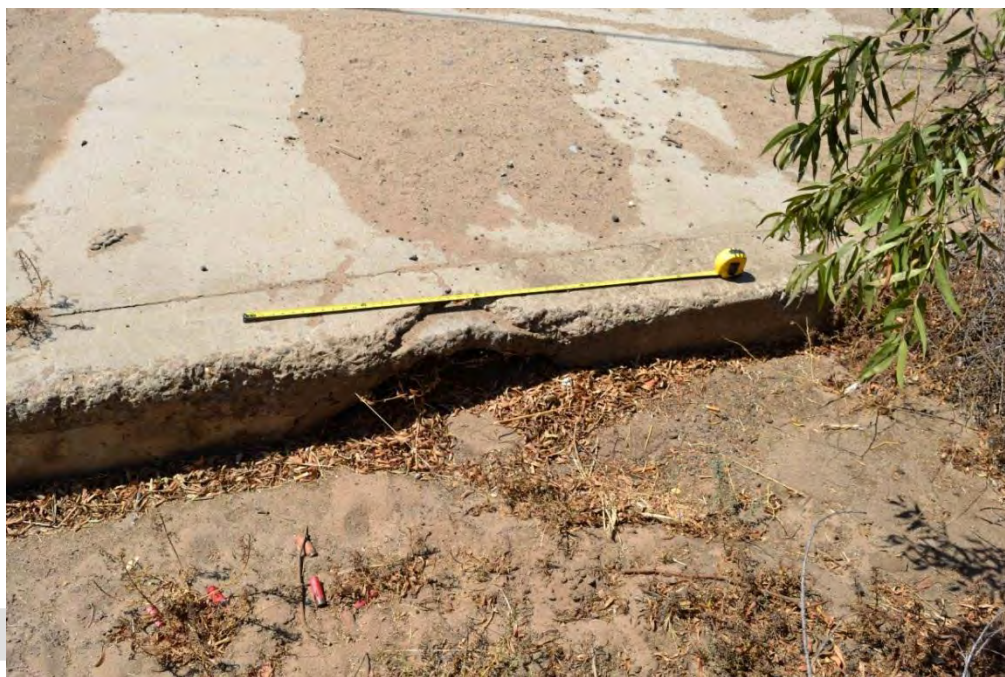
Figure 3. Looking west from HCWA. Note 3 foot diameter pipes almost entirely buried in sediment.
