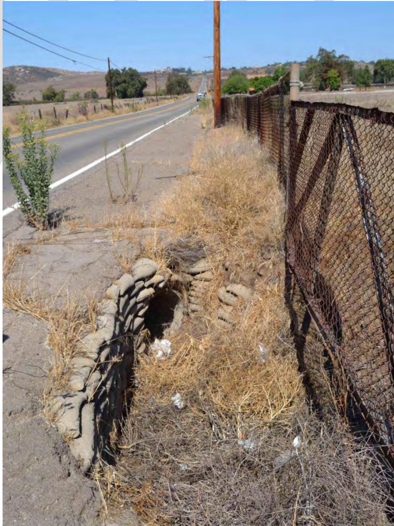
Figure 7. Looking north towards Rancho Jamul Road.
