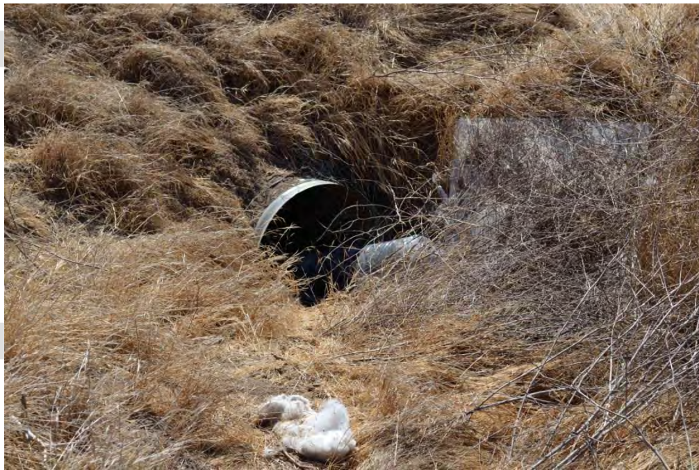
Figure 13. Looking east at culvert set eight feet below road surface
