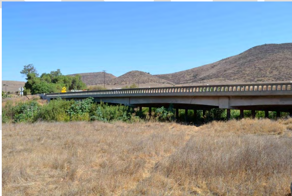
Figure 19. Looking east from RJER towards HCWA
