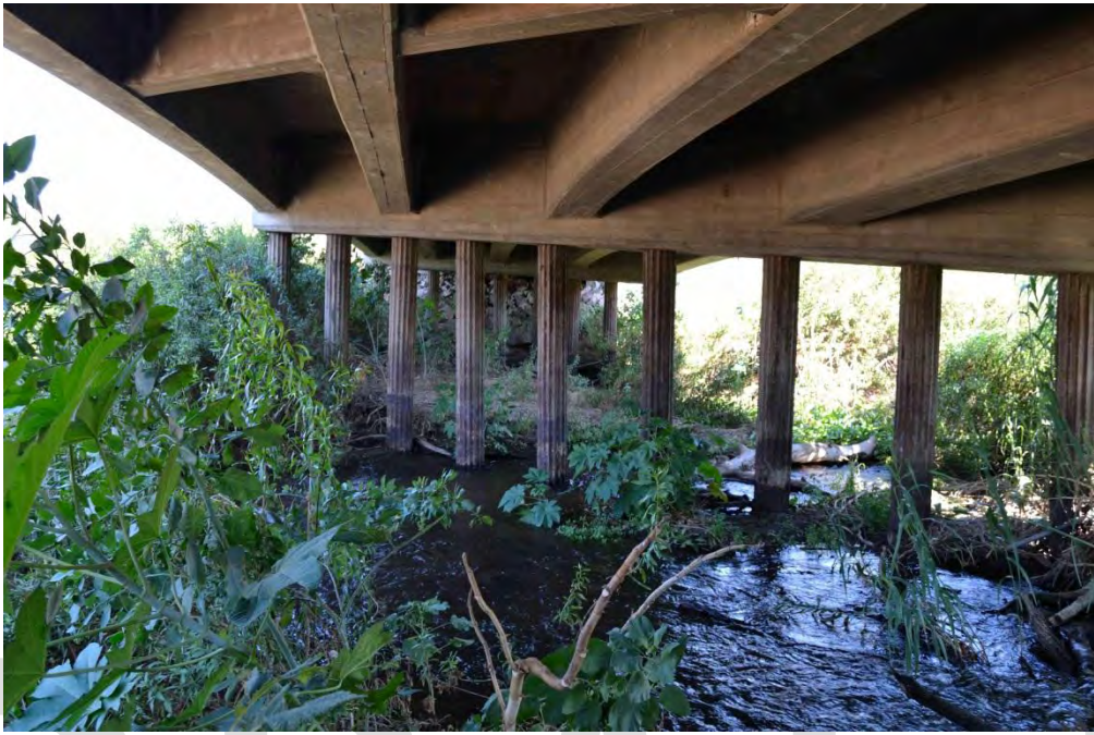
Figure 20. Looking north from south end of bridge
