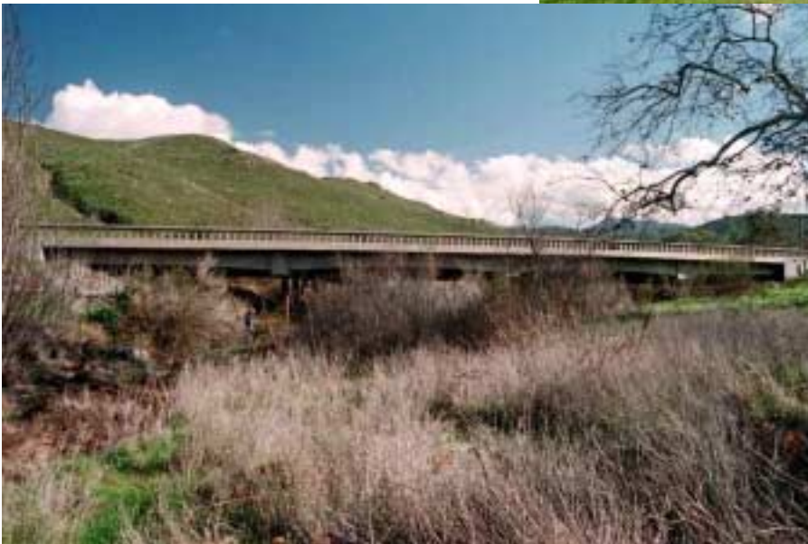
SR-94 bridge over Dulzura Creek, looking east from downstream side.
