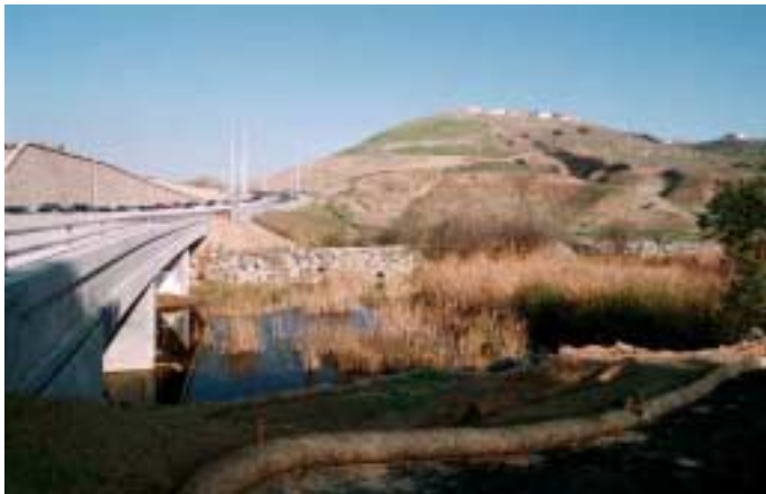
Vista Sorrento Pkwy bridge over Peñasquitos Creek looking north.
