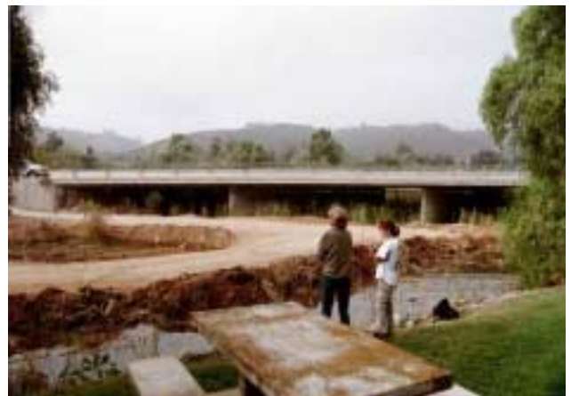
Sorrento Valley Rd bridge over Peñasquitos Creek looking west.
