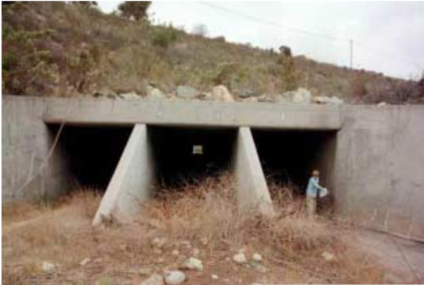
O'Neal Canyon culverts under Alta Rd looking northwest (downstream).
