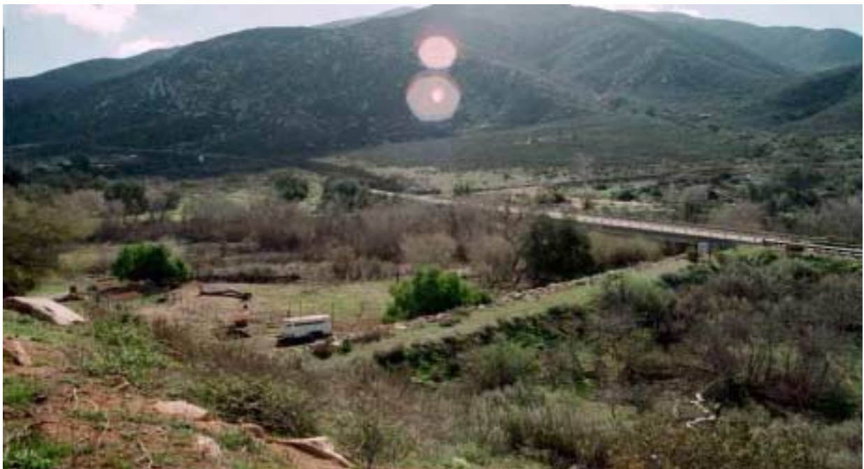
SR-94 bridge over Cottonwood Creek looking south from north and east side of bridge.
