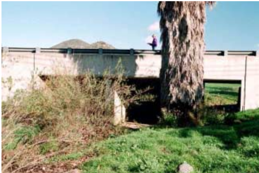
SR-94 bridge over Jamul Creek, looking north.
