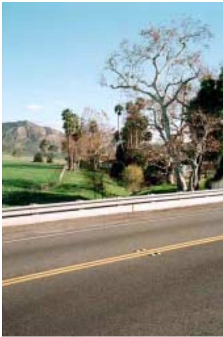
Looking north up Jamul Creek from SR-94 bridge.
