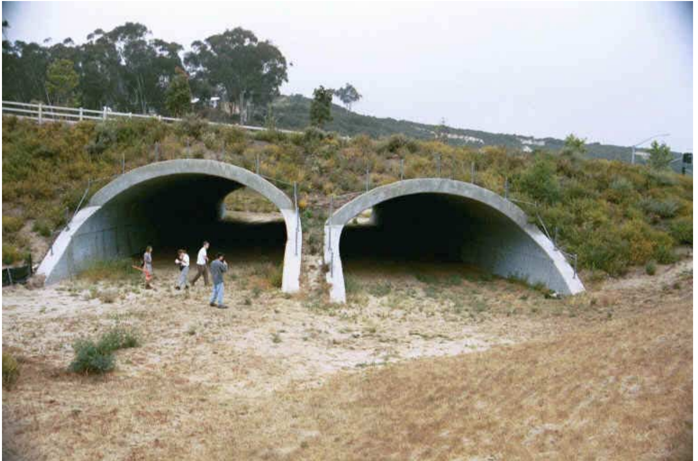
Culverts under Carmel Country Rd in lower Shaw Valley looking west.
