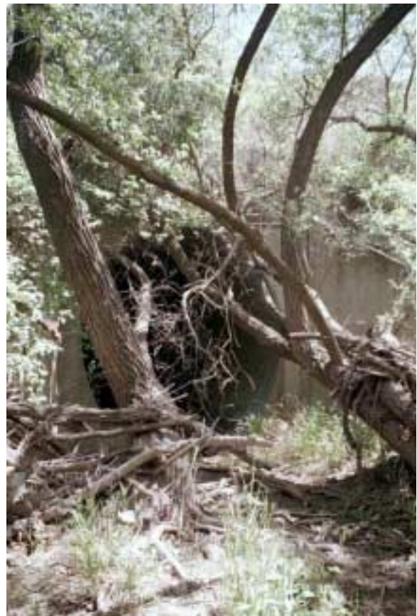
Chocolate Creek culvert under Peutz Valley Rd, looking north.
