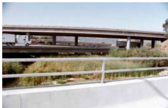
I-5/805 merge bridges, looking west from Vista Sorrento Pkwy bridge.
