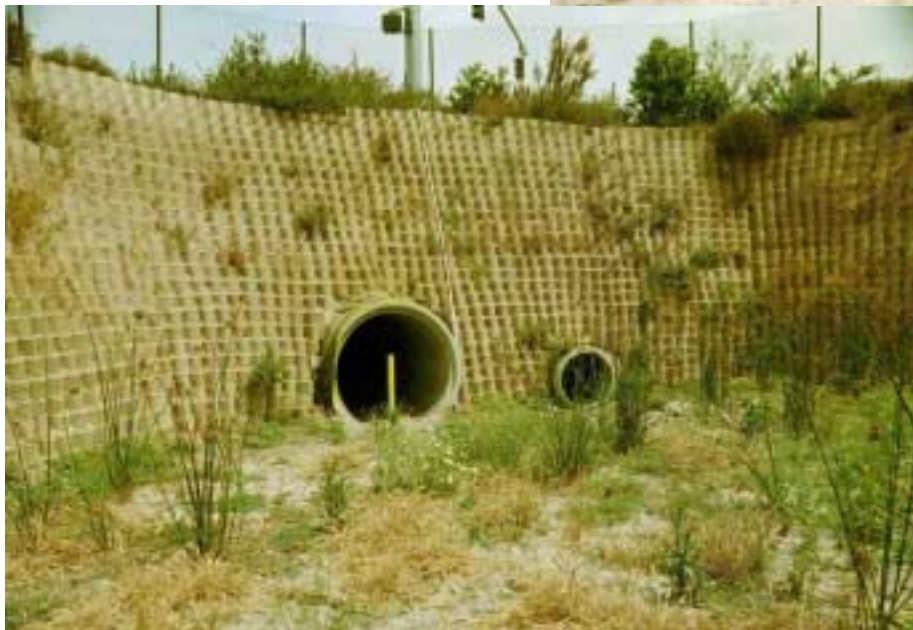
Culvert under Otay Mesa Rd from the south side looking north.
