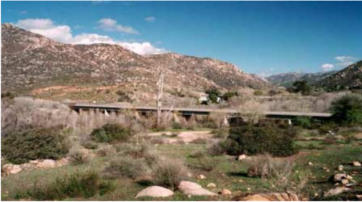
SR-94 bridge over Cottonwood Creek looking north from south and west side of bridge.
