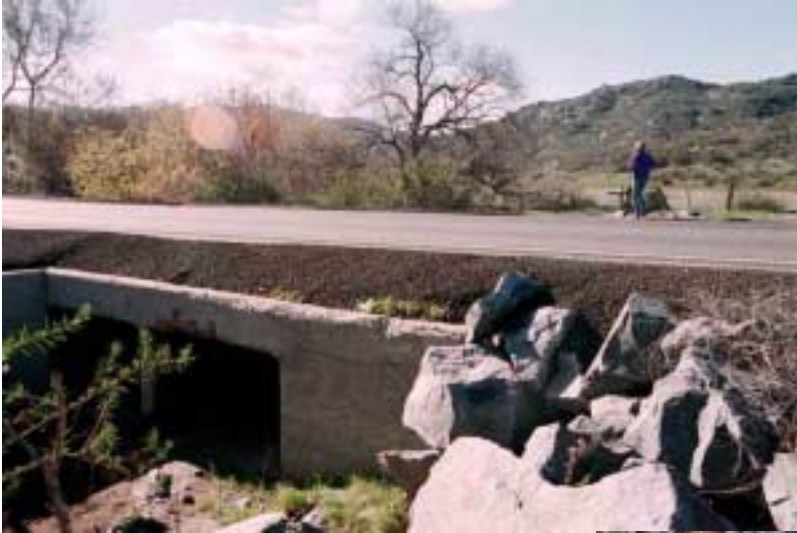
Hollenbeck Canyon drainage culvert under SR-94 looking south.
