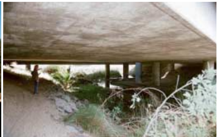
Vista Sorrento Pkwy bridge over Peñasquitos Creek looking east.
