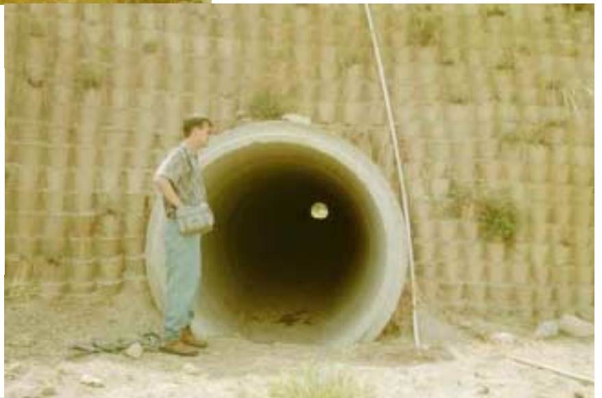
Culvert under Otay Mesa Rd from the south side looking north.
