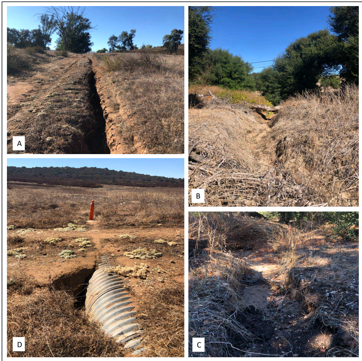
Figure B-10. Erosion on the Montecito Ranch Preserve. A. Erosion (gully) on road edge. B. and C. Erosion in drainage paralleling SR-78. D. Erosion in road associated with culvert.
